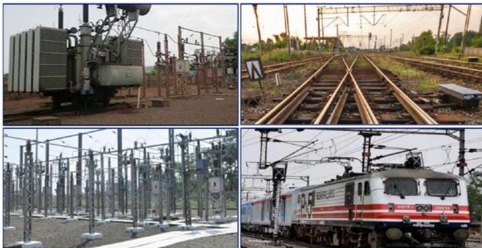
Fig 148: Texmaco’s Infra – Electrical Division projects
